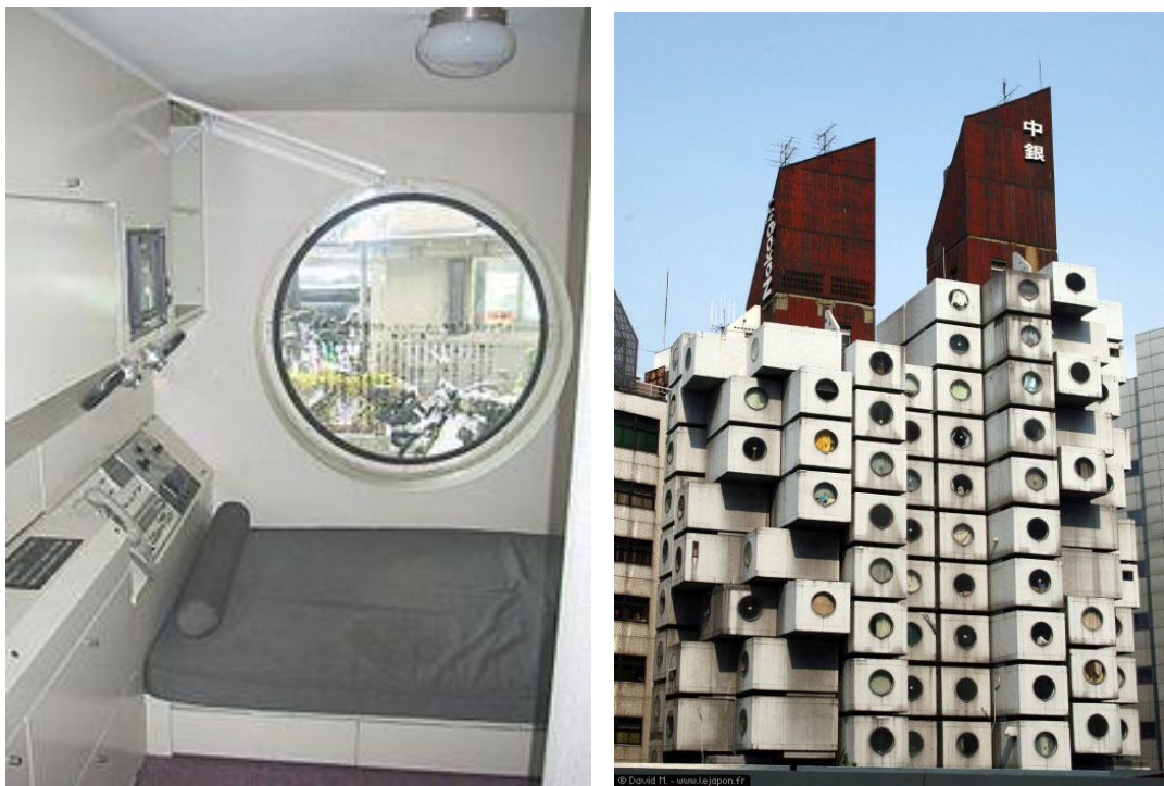
Fig. 1: Nakagin Capsule Tower designed by Kisho Kurokawa and completed in 1972. The photo on the left shows the interior of a single residential capsule and demonstrates the efficient use of compact space. The photo on the right demonstrates the unique structure of the building and clearly shows the permanent red towers as well as the more temporary pods that surround them.
