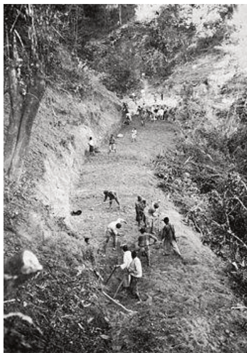
Figure 5: Construction of the Burma Road
