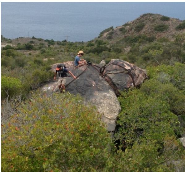
Figure 5. Large block of competent amphibolite. Softer weathering bed rock around it probably is serpentinite.
