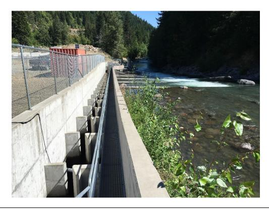
Figure 4: Fish ladder located on the Hood River in Oregon, allowing salmon passage around a small obstruction in the main channel of the river. Water flows down the channel, but its flow is slowed by the concrete barriers. Such structures can help fish navigate smaller obstacles but are often not feasible options for allowing passage around larger dams.
