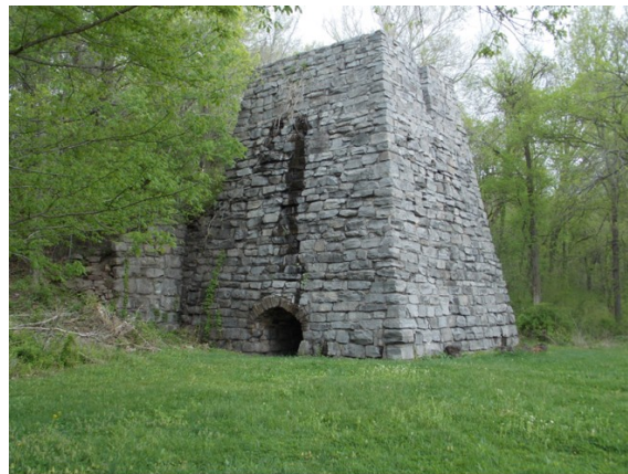
Figure 19. Reconstructed historic iron furnace in Shawnee National Forest, Illinois. Credit: Hidden Springs Ranger District.
