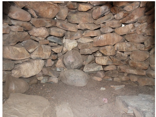
Figure 15. Interior of Crestone Hut #4, showing the corbelled construction style.
