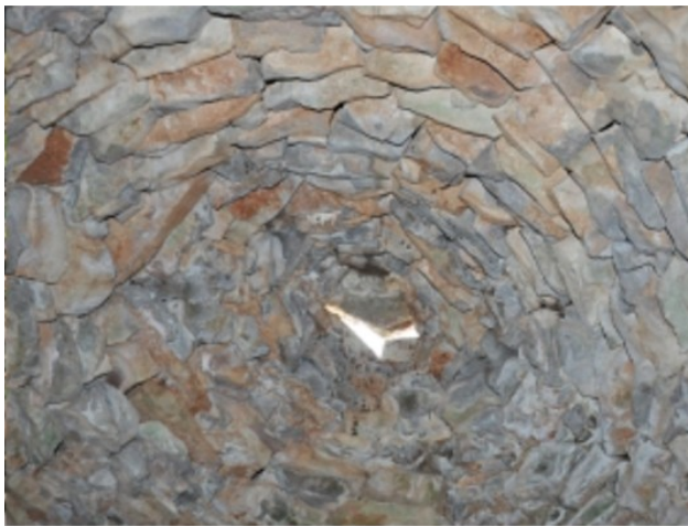
Figure 14. Interior of a trulli , showing the corbelled construction style. Credit: Miosi (2018:219).
