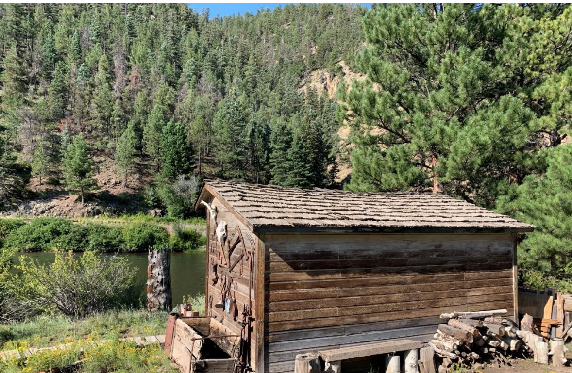
Figure 1. The waiting shed in its current location on the Marvel property in South Fork, Colorado. Across the Rio Grande River in this photograph was the original Alamosa-Creede track (southern aspect).
