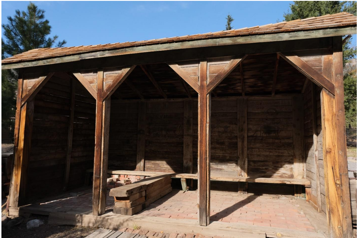
Figure 17. View of the southern entryway of the waiting shed showing the wooden post that demarcates the different entrances and the triangular braces. The original wooden bench is included in this photograph and spans the entire length of the northern interior wall (northern aspect).
