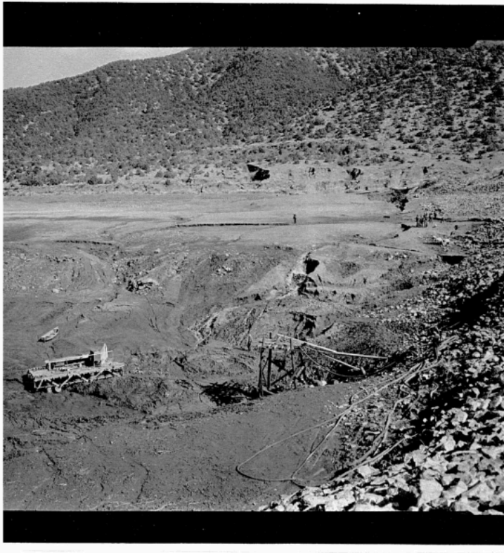
Figure 2.2 Cleaning out Two Mile Dam and Reservoir. Unknown Date (Post 1904 flood?) Source: Fray Angélico Chávez History Library
