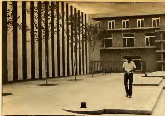
The recently completed Packard Arts Center is open for classes despite some superficial cracks on the West wall.
