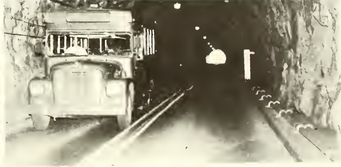
An Air Force bus heads down the main tunnel leading to the North American Air Defense Command's Combat Operations Center deep within Cheyenne Mountain.
