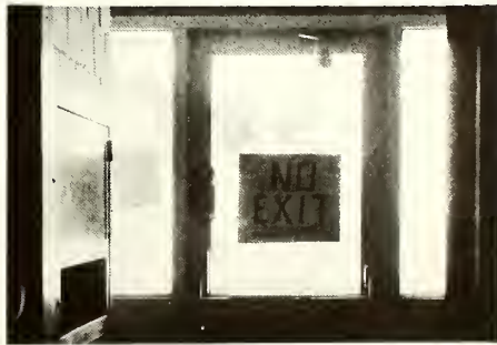
ONE OF THE NEW FIRE DOORS installed in Slocum Hall in an attempt to keep unwanted visitors out.
