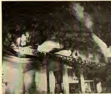
SMOKE POURS from flaming Arthur House as firemen fight blaze.
