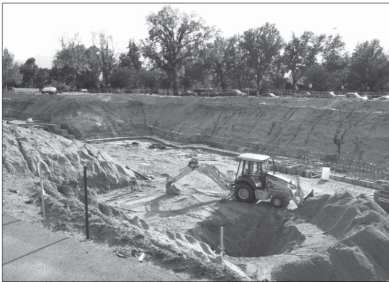
Bulldozers work to clear space for the new Cornerstone Arts Center.
