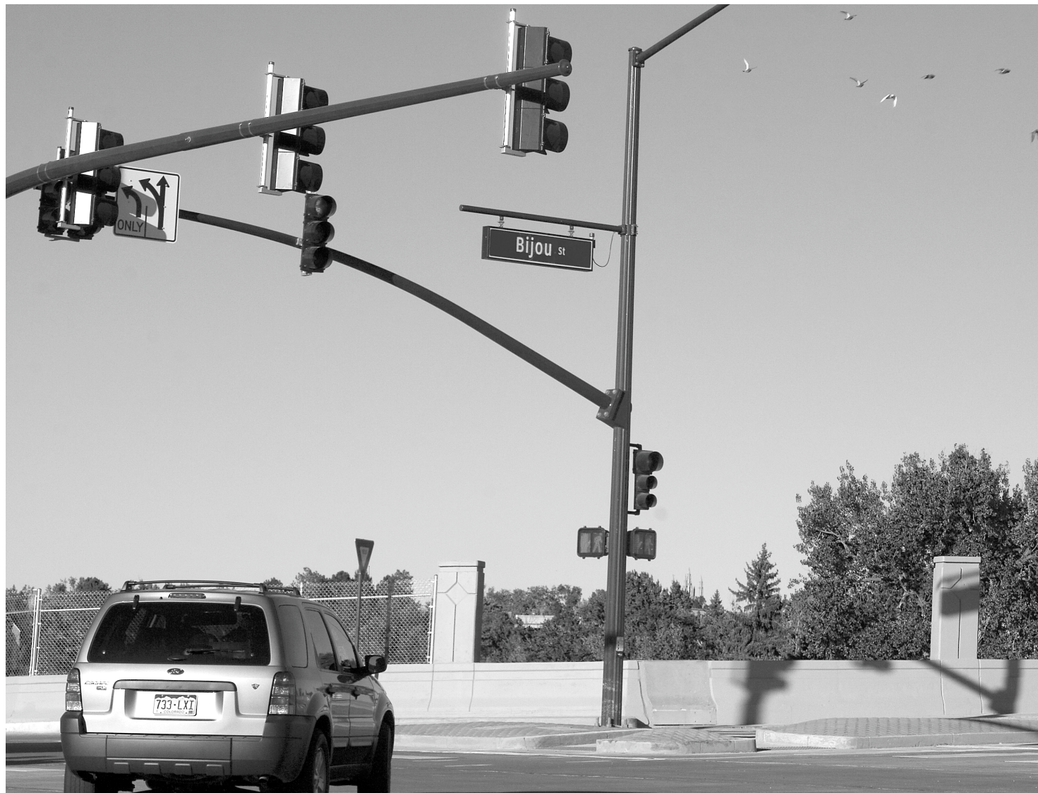
Since its completion on October 1, the Bijou Street Bridge once again serves as Colorado Springs' artery into downtown.
