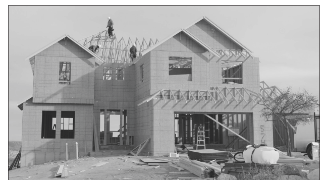
A home is rebuilt after the fire. Photo by Brendan Young.
